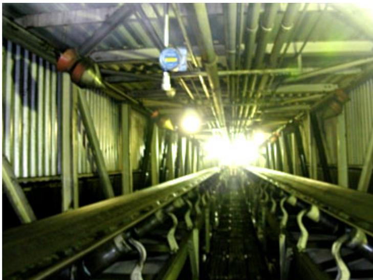
*fig. 6 - Looking down the main conveyor structure. A CO monitor located above and left of center. Two conveyor belts on either side, redundant to minimize the potential of shutting down the plant if a single conveyor shuts down.*
