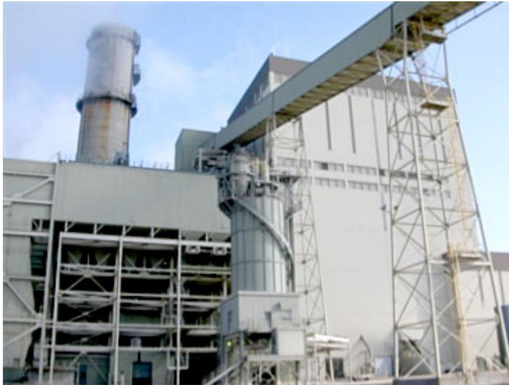
*fig. 7 - A view of the main conveyor as it heads into the power plant building. The top of the building is about 13 stories high.*
