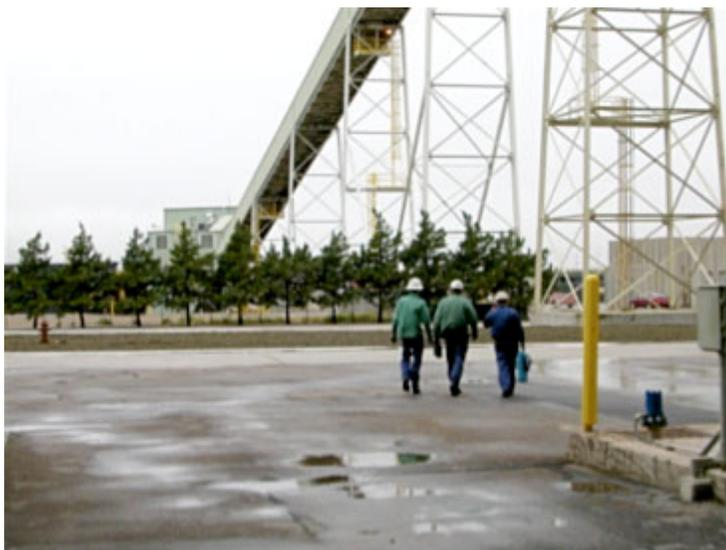
*fig. 3 - The main conveyor structure at Harrington rises from the crusher building behind the trees. The live pile, car dump, and reclaim tunnel are located on the far side of the crusher building. The walls and floors are corrugated metal and there are numerous openings in the structure.*
