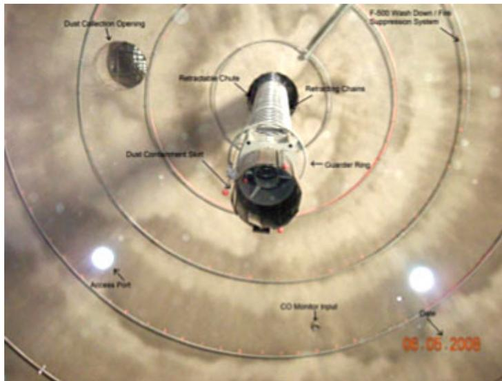
**fig. 13 - The inside of a dome showing the various components and their purposes**
