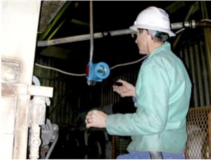
*fig. 4 - A CO monitor undergoing calibration during initial installation at the top of the conveyor structure*
