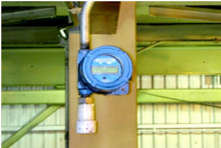
*fig. 5 - Typical CO monitor installed along a belt head drive location. Note the white cap on the sensor head. This is the splash guard used to prevent wash-down work from loading the sensor with water.*
