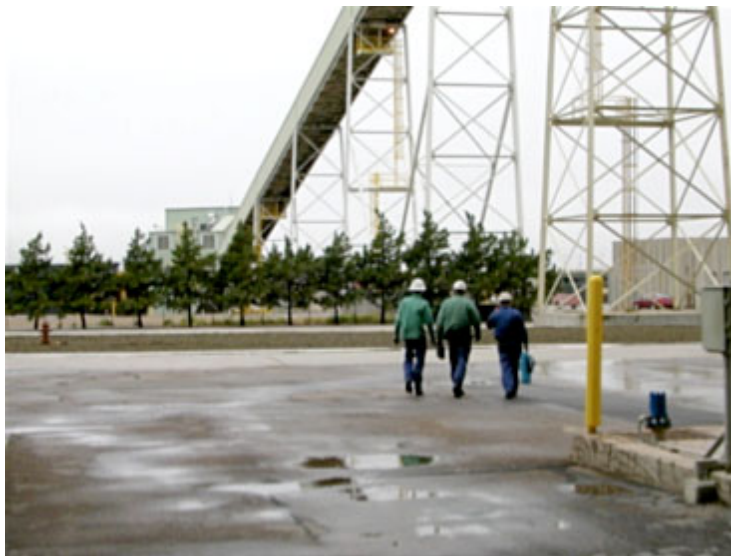
fig. 3 - The main conveyor structure at Harrington rises from the crusher building behind the trees. The live pile, car dump, and reclaim tunnel are located on the far side of the crusher building. The walls and floors are corrugated metal and there are numerous openings in the structure.
